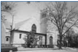
38 25 E. Benton Ave. First Congregational United Church of Christ 1905-06 M.J. Morehouse, Architect
