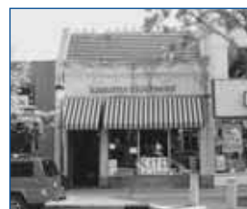
9 28 W. Jefferson Ave. NHS Western United Gas and Electric Co. 1906; remodeled 1932
