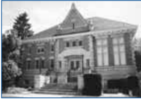
42 110 S. Washington St. Nichols Library 1897 M.E. Bell, Architect
