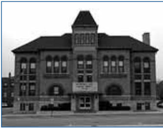
24 5 N. Ellsworth St. SS. Peter and Paul Grade School Wenker Hall 1892
