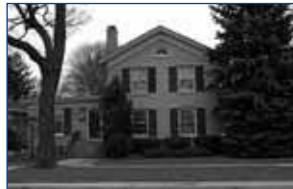
Ellsworth St. entrance
