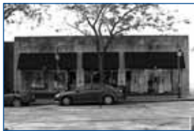
4 223 S. Main St. 1930s Commercial Deco Facade
