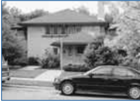
17 48 E. Jefferson Ave. NHS Dr. Ruliff L. Truitt Residence 1916 Harry Robinson, Architect
