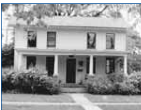
32 154 N. Center St. NHS David Frost Residence 1868
