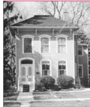
19 429 E. North Ave. Sucher/Dudley House c. 1871
