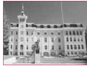
31 30 N. Brainard St. NHS Old Main 1870; south wing added 1890 John Van Osdel, Architect
